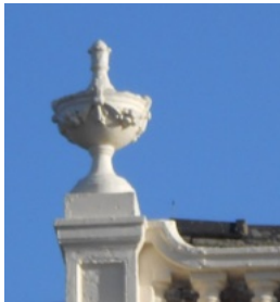
Anchor House detail.
